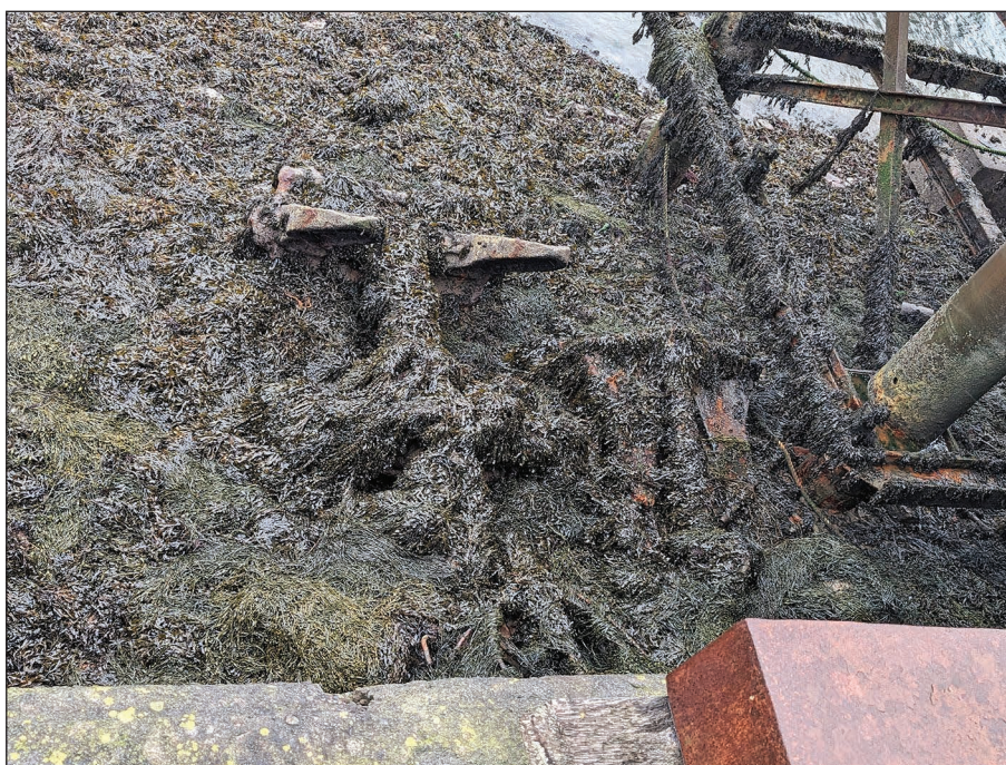
Figure 11: Anchors 1005 and other debris along western side of Western Wharf
