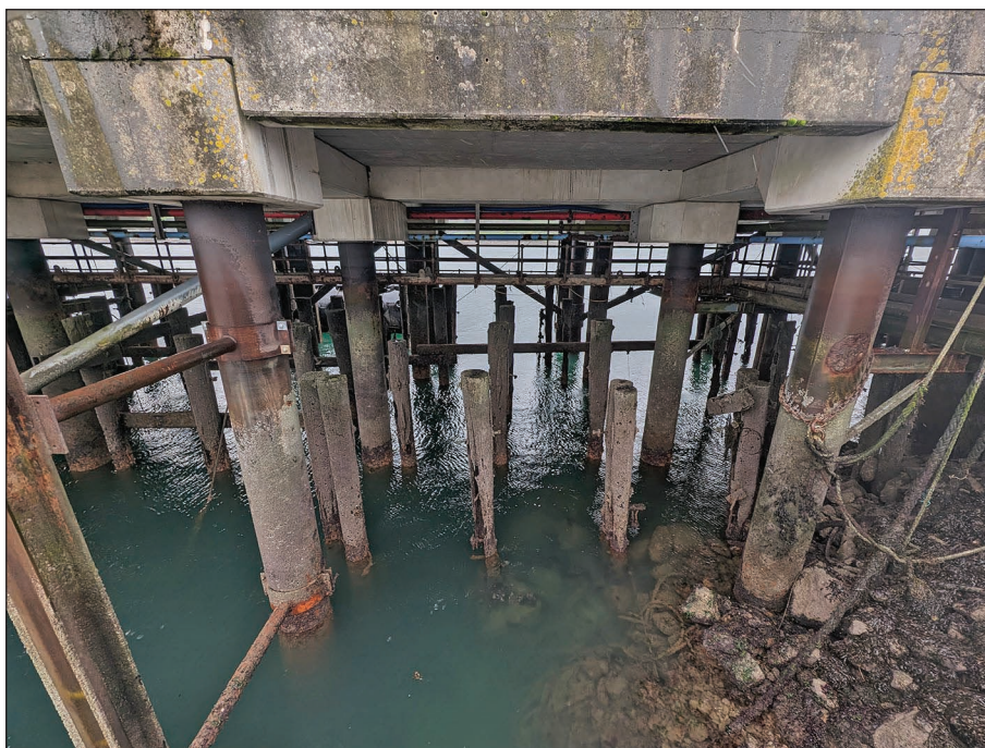
Figure 12: Original timber construction of Queen's Wharf below modern replacement
